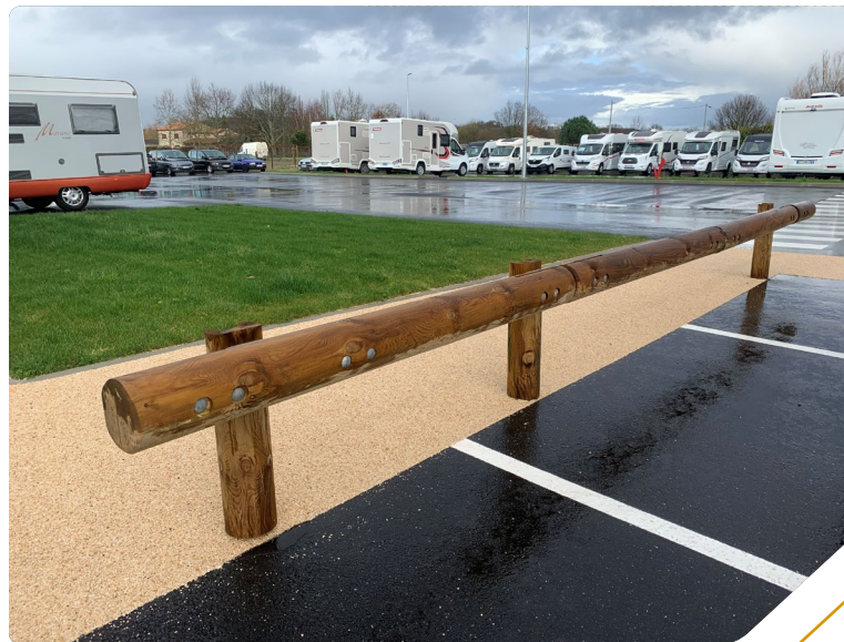
Parking de surface commerciale
